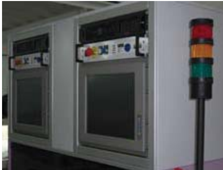
Independent IPC, UPS, Monitor and Power management unit per station module
